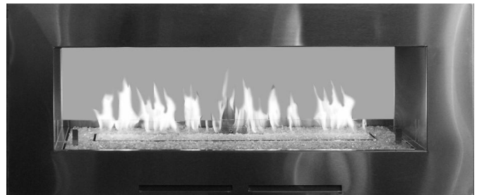
Figure 8 - Correct Burner Flame Pattern
