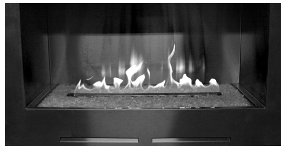
Figure 9 - Incorrect Burner Flame Pattern caused by port blockage
