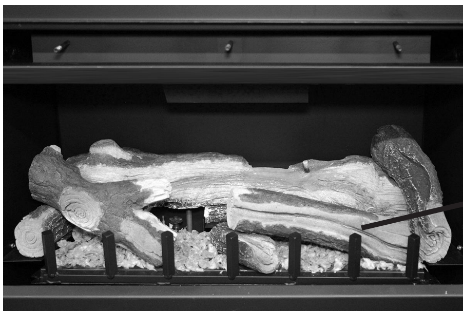
Figure 22 - Installing Right Upper Log #6
