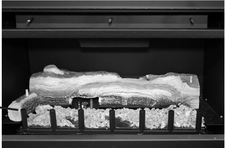
Figure 18 - Installing Left Base Log #2
