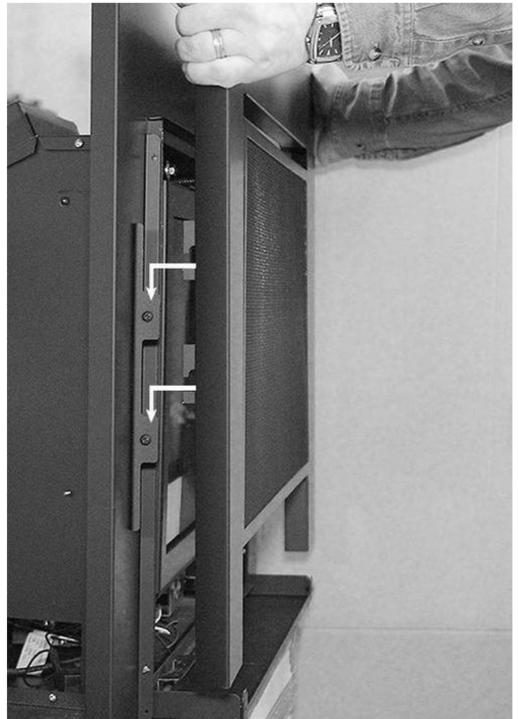
Figure 26 - Installing Outer Face
