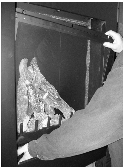
Figure 36 - Removing Glass Frame
