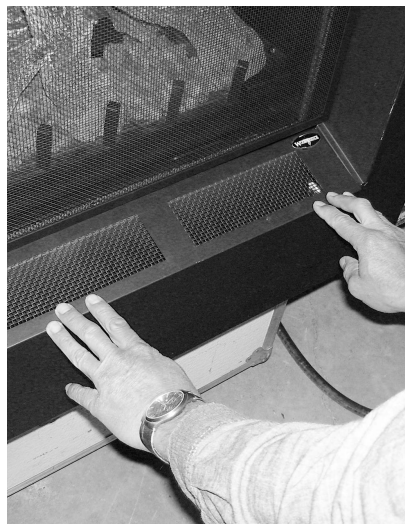
STEP 6: Tilt the Panel down to rest on the face support.
