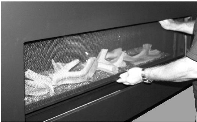
STEP 3: Position the safety screen inside of the fireplace in front of the glass door. Locate the two small vertical studs along the glass door frame bracket.
