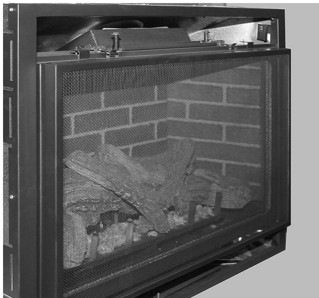
STEP 4: Make sure the safety screen is securely positioned on the studs.
